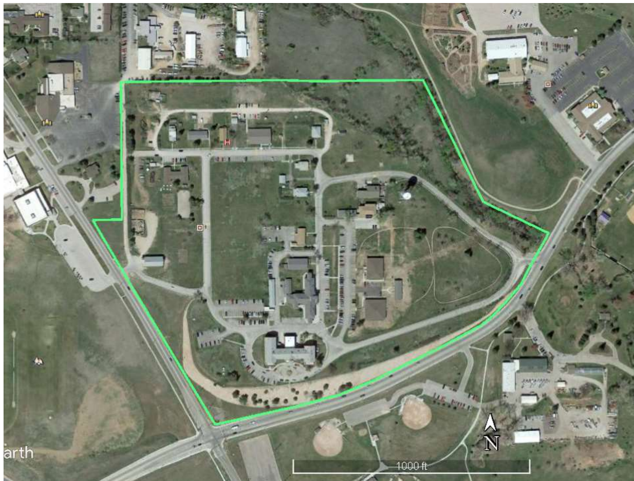
Figure 1. The Area of Potential Effects for the Rapid City IHS Health Center undertaking.
