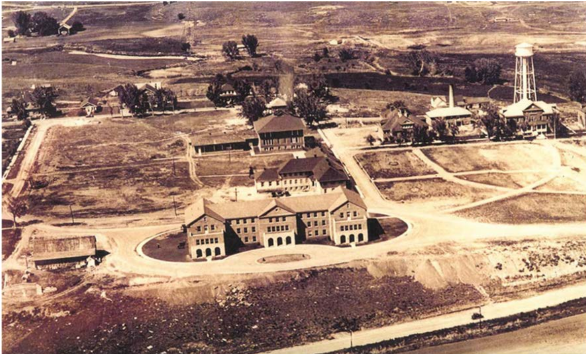
Figure 3-1. Circa 1939-1940 aerial photo showing renovation work at Sioux San.
